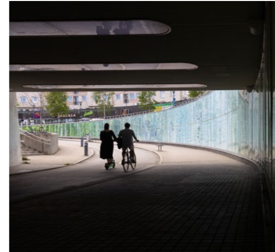
A central underpass was widened and made lighter for safety Credit: Fredrik Larsson
